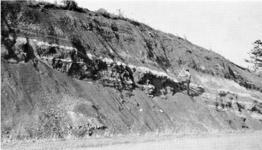
FIG. 4.—Road cut through the Lower Carboniferous formation near Kingsclear, N.B. The white streaks are light greenish colored gypsum rocks, while the dark coloured material consists of bright red mud-stone, containing often as much as 80 per cent calcium carbonate.
