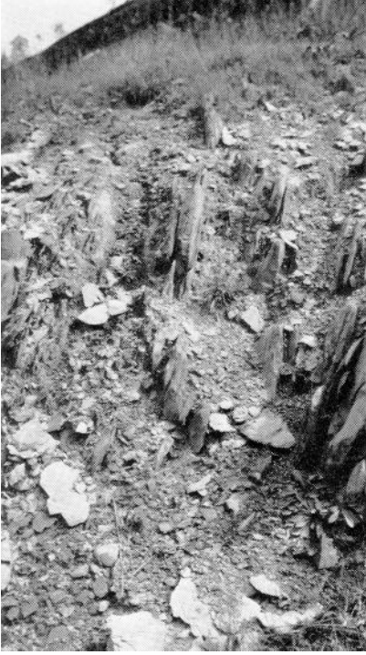
FIG. 2.—Exposed rock of Pre-Carboniferous formation. The weathered rock is very soft and crumbly. Note the steep incline of the unweathered rock which provides good drainage.
